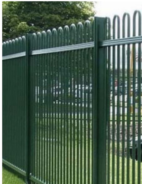
Security fence 2.4m high bow top fencing
