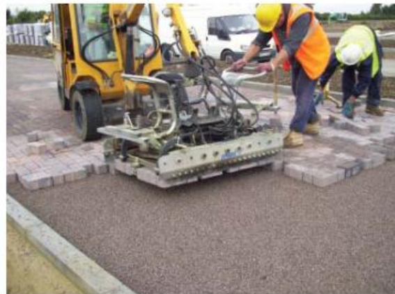
Permeable block paving being machine laid in Cambridgeshire
